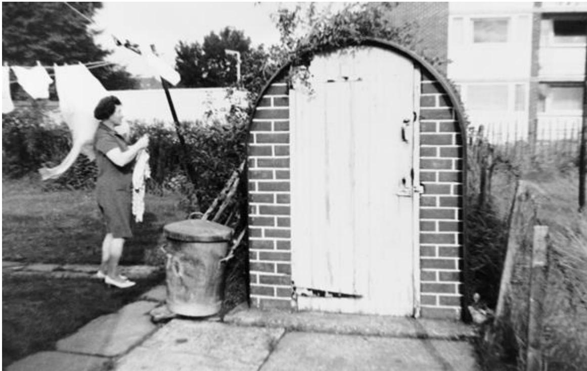
*A garden shelter during the war. The Anderson shelter seen here, designed by the engineer David Anderson, was supposed to be installed below ground level, but in areas with the risk of flooding this was difficult to do. They were no defence against a direct or near direct hit. (Courtesy of the Imperial War Museum)*
